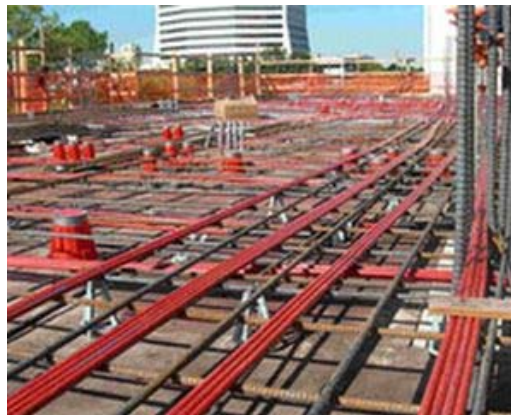
Figure 6 – Two-way post-tensioned floor system ( www.suncoast-pt.com )
